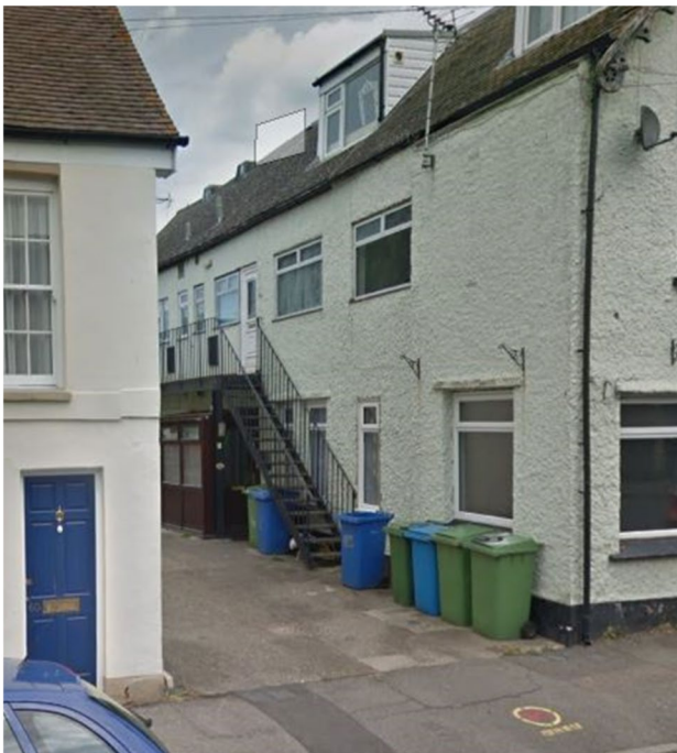
Similar steel staircase in the High street
